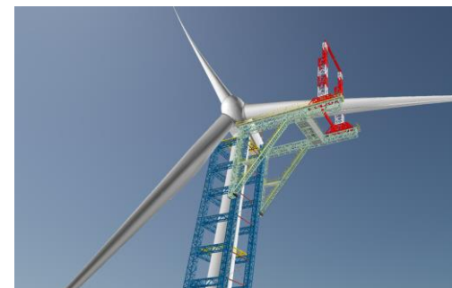
Wind-blade-install construction method
