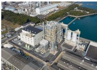
Biomass power plant
