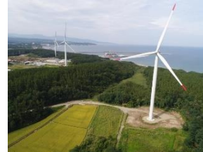
Shichiri-nagahama Wind Farm
