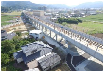
Kyushu Shinkansen Ureshino Overpass
