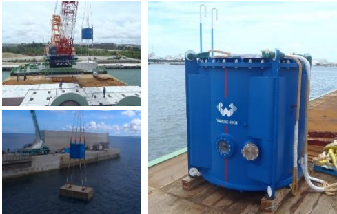
Underwater Gyro that controls suspended load rotation
