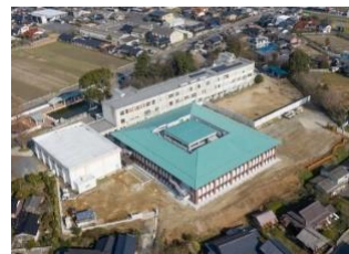
Elementary school building
