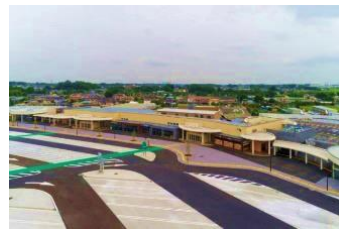
Expressway service area facilities
