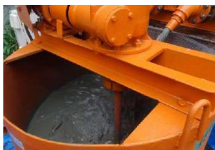
(a)基材練混ぜ状況
