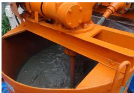
(a)基材練混ぜ状況
